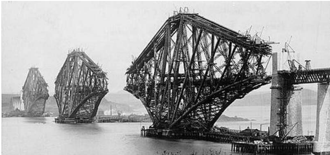
Forth Bridge under construction, c1888
